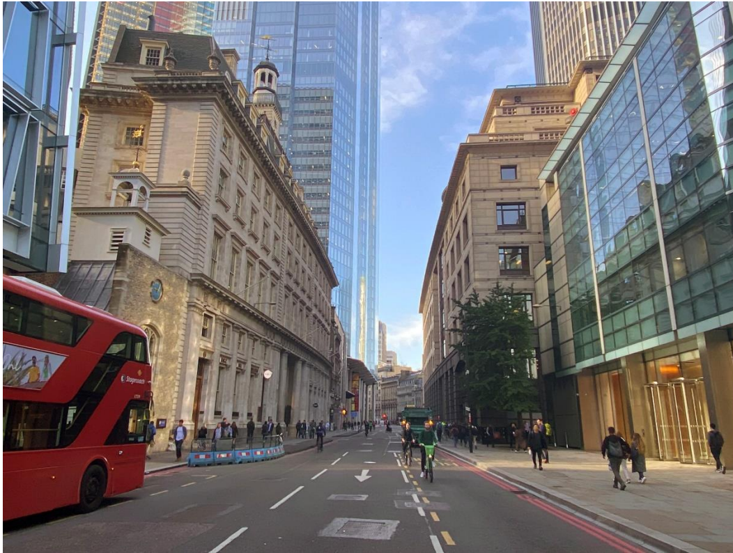
Image 7: East elevation of and entrance to existing building (right)
