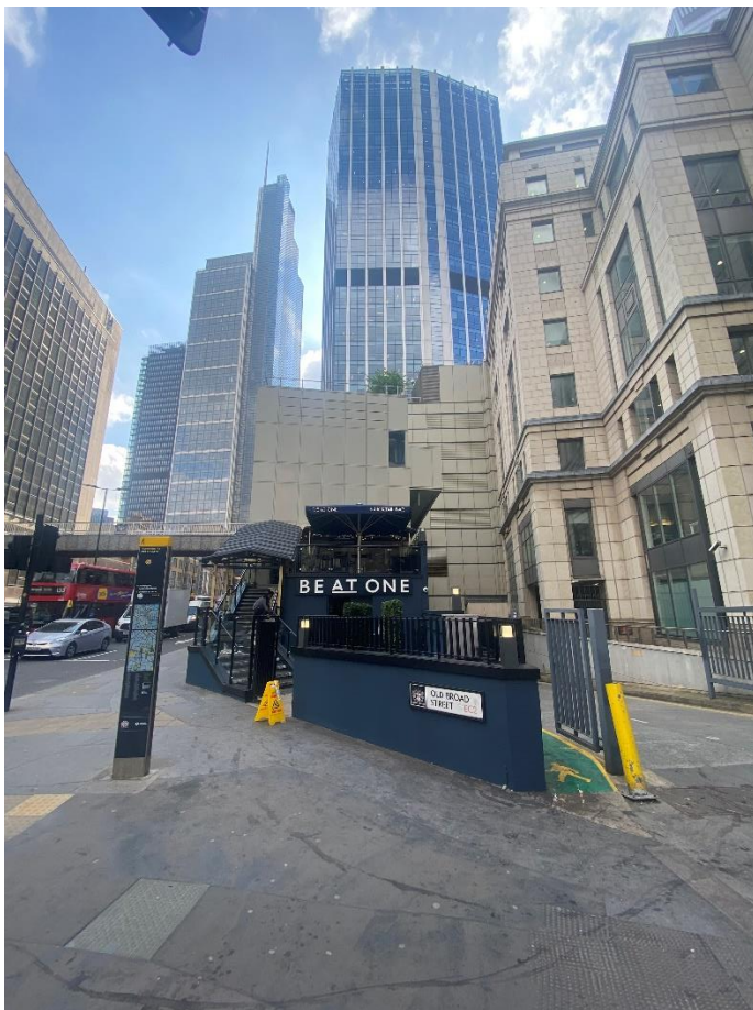
Image 8: West elevation of existing building with servicing ramp from Old Broad Street
