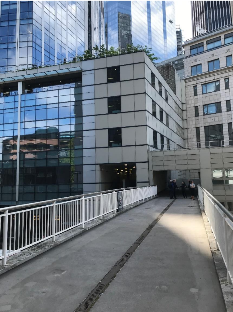
Image 5: City Walkway Bridge into existing site
